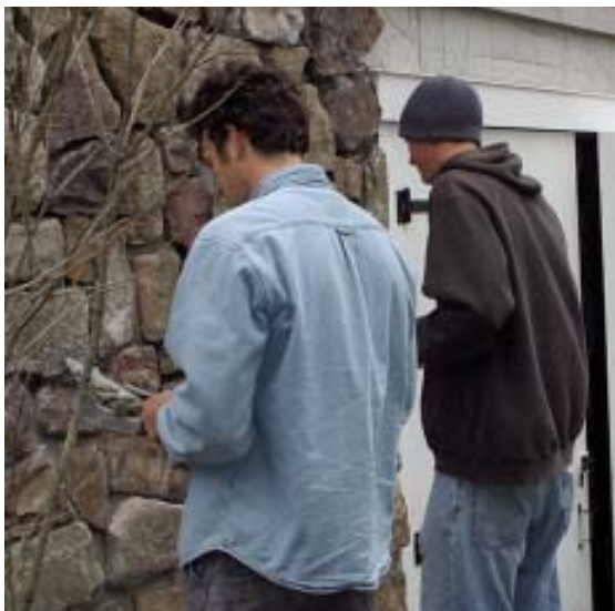
Figure 4. Periodic jointing of the stone provided support between courses to prevent slippage before the mortar set up.
