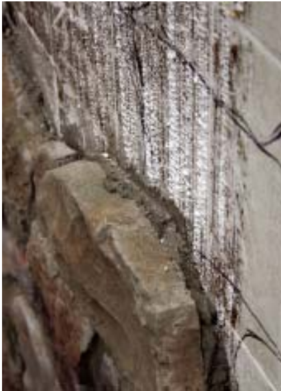
Figure 3. To ensure a void-free bond, the author applied mortar to both wall and stone a piece at a time and removed the squeeze-out. While the abrasion marks seen on the foam here are not essential for bonding to expanded polystyrene, roughening the surface of smooth-faced extruded polystyrene foam would definitely be a good idea.
