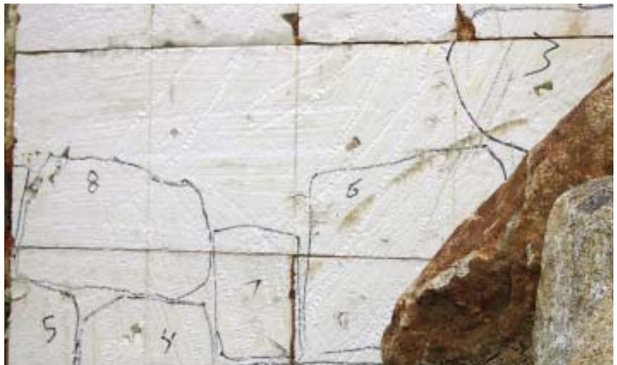
Figure 2. Once the pattern was determined, the layout was traced on the wall and each stone numbered for reference.
