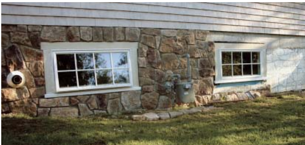
Figure 1. Dry layout allowed the installation crew to plan a natural-looking pattern that involved minimal cutting. Stones with a slight taper along one edge were chosen to tuck under the wood siding at the top of the foundation.
