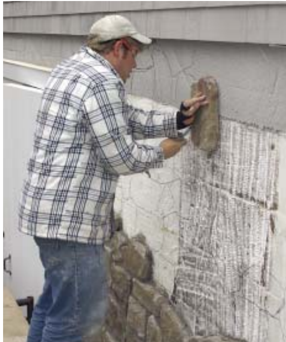
Figure 2. Once the pattern was determined, the layout was traced on the wall and each stone numbered for reference.
