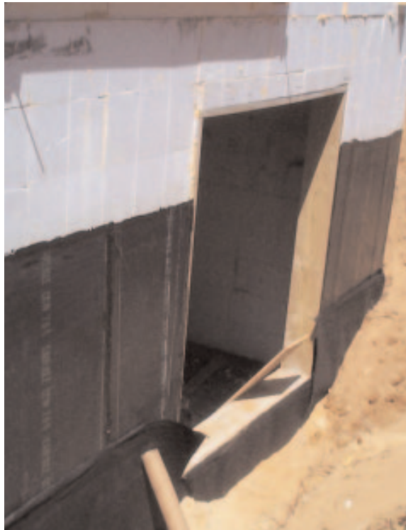
Figure 3. Where the membrane meets door or window buck, special flashing tape (not yet installed in photo) seals the transition into the opening.
