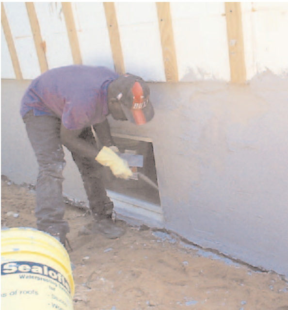
Figure 8. Using a stainless steel trowel prevents rust stains in stucco.
