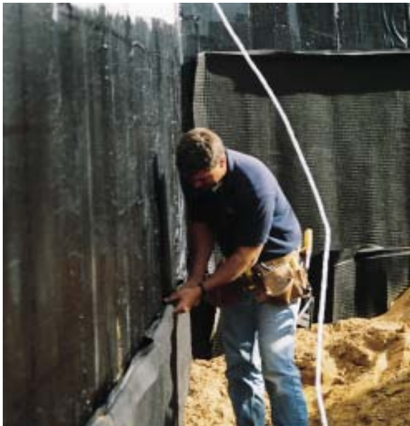
Figure 7. Backfill pressure holds the drainage mat firmly in place. Stucco protects the exposed portion of the ICF foundation, and covers the upper edge of the membrane.
